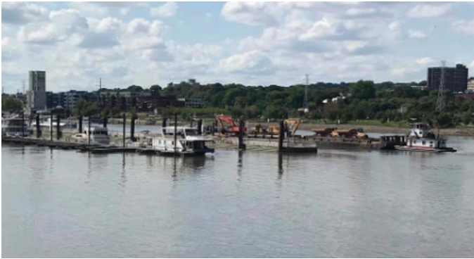
Dredging of the Lower Harbor (September 2018)
